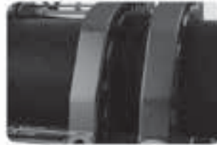
5. remove heater plate , close clamps to bring bead up .
